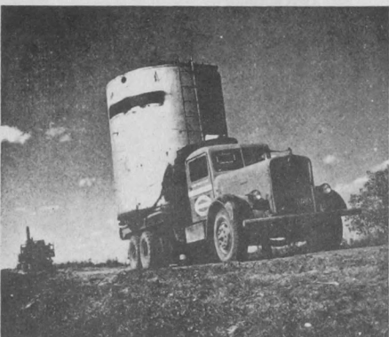
12 With new and improved roads it was possible to transport to the field such heavy equipment as storage tanks that were already rivetted and to set them up to store crude
